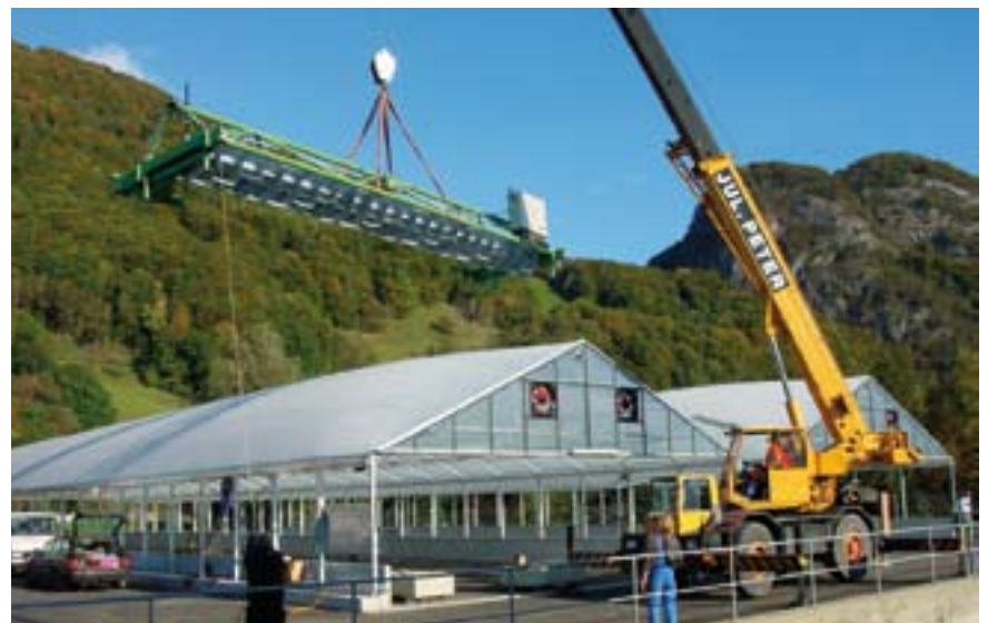
Montage Klärschlamm-trocknungsanlage [Schweiz] Sewage drying facility installation in Switzerland
